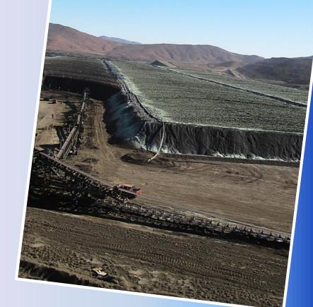
Heap Leaching Drip Irrigation System
